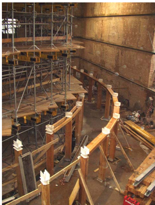
Separated wooden structure inside the Cavea 's brick walls
